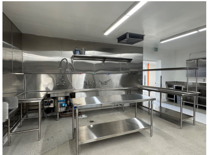
Almost complete: the new, very shiny main sink area
